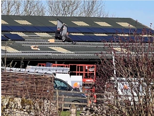
PV Panel installation.
