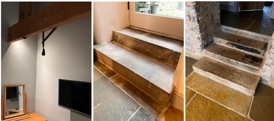
Retained milking equipment in The Milking Parlour, and re-used stones reclaimed from elsewhere in the properties and used as steps.
